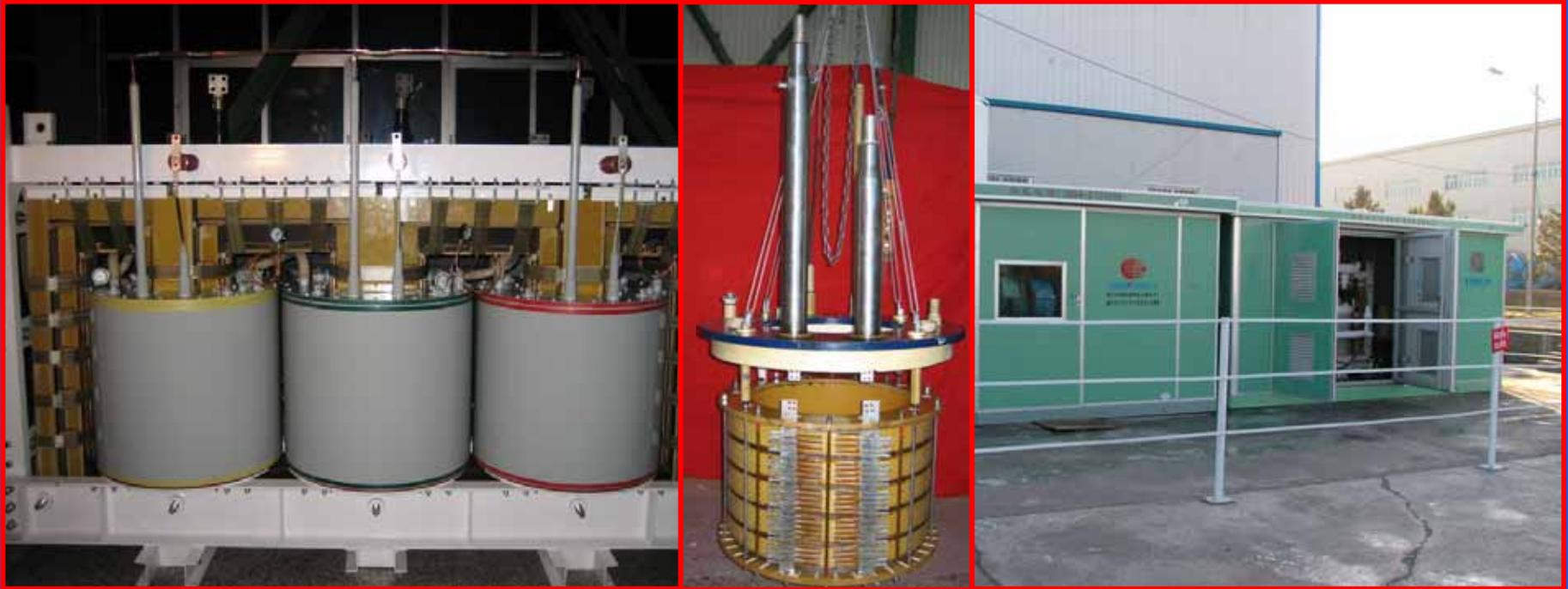
The 630kVA/10.5kV/0.4kV HTS power transformer was installed at the headquarters of TBEA in Changji City, Xinjiang Autonomous Region, and was energized on November 21, 2005.
