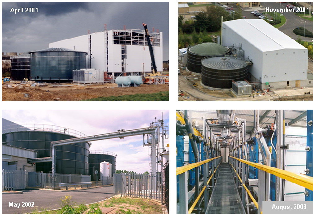
Figure 11-7 Progress With Regenesys Construction at Little Barford Generating Station
