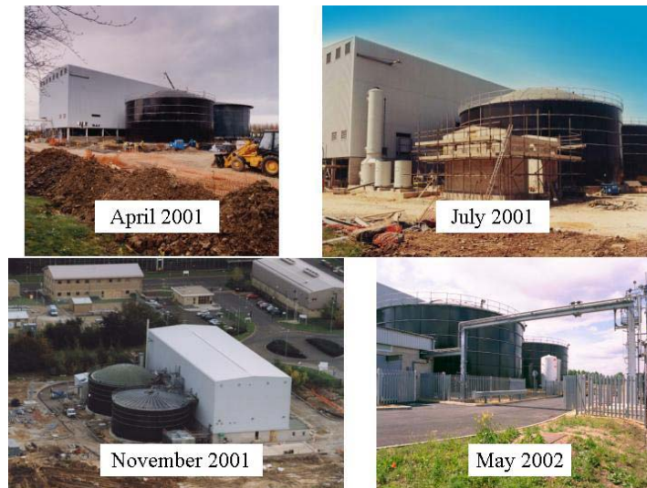
Figure 7 Progress with Regenesys Construction at Little Barford Generating Station
