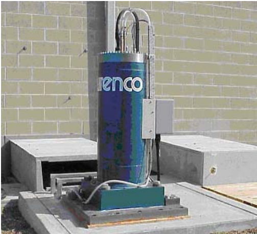
Figure 5 High-Speed Vertical-Shaft Composite Power Flywheel
