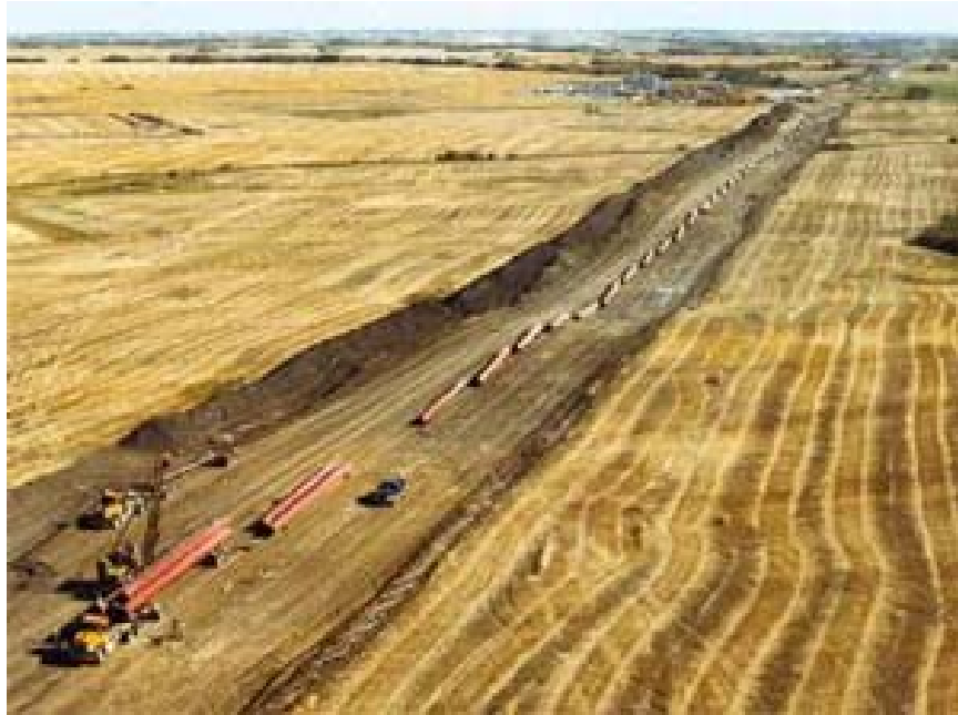
Figure 8-2 Example of gas pipeline being delivered to site in preparation for welding
