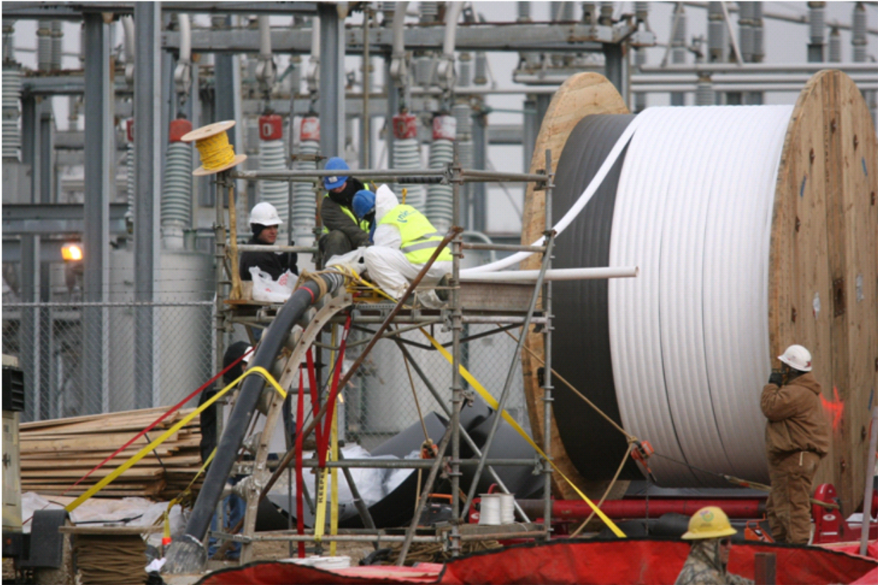
Figure 8-11 Cable pull for a superconducting cable
