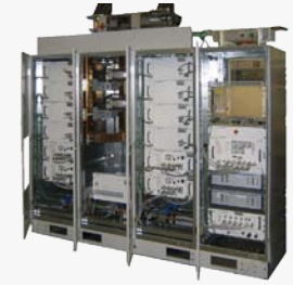
In tunnel alcoves
