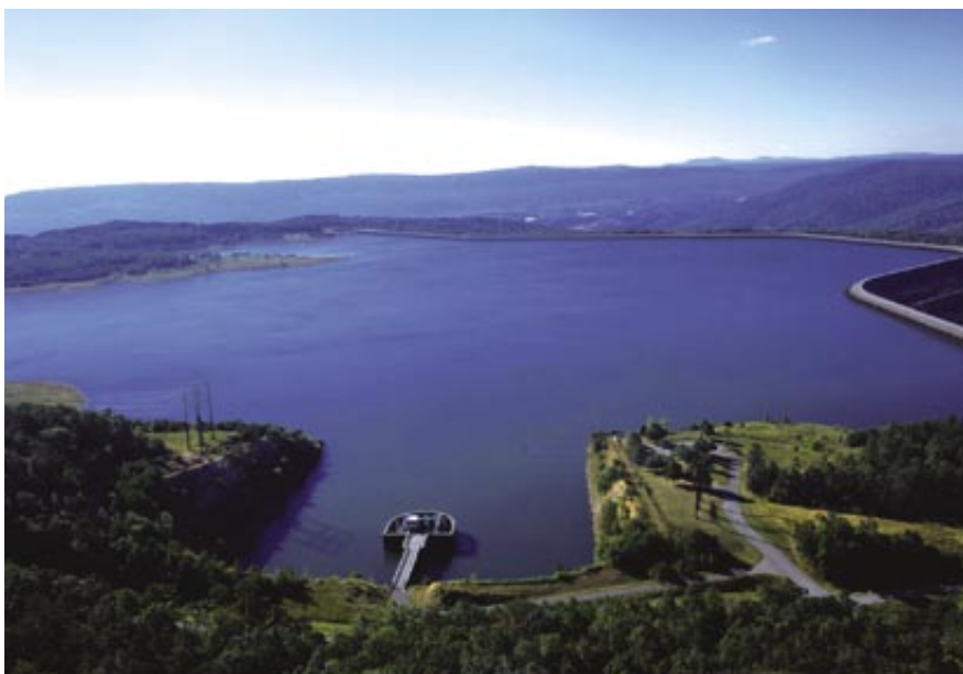
PUMP-FILLED LAKE atop Raccoon Mountain in Tennessee stores enough potential energy to create 32 gigawatt-hours of electricity when drained through its hydroelectric dam. Every 70 kilometers of SuperCable would store an equivalent amount of energy in the form of hydrogen.
