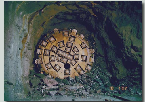
Cutter Head of State-of-the-Art Tunneling Machine (photo courtesy E. Cording, University of Illinois-UC)
