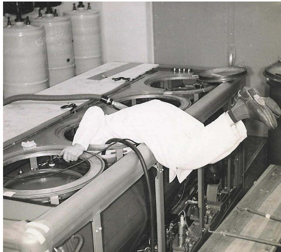
Anode Porcelains & Mercury Cathode Tank
