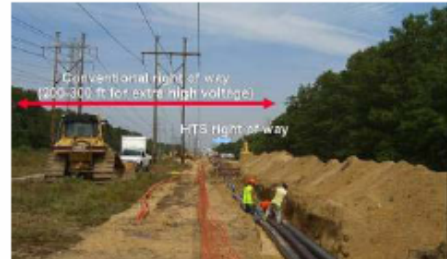
Long Island Power Authority HTS Cable Project (September 2006)
