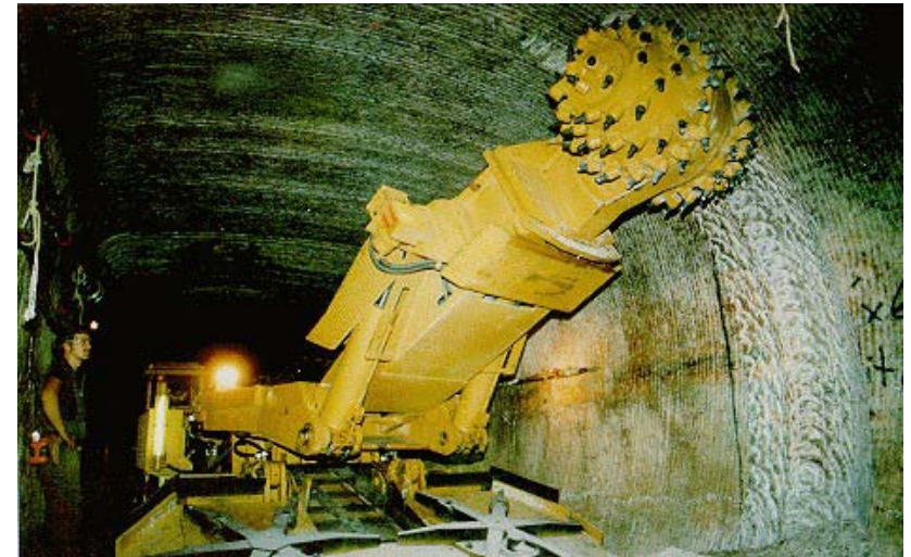
Alpine miner dressing out a tunnel mined by a drum road-header in the WIPP facility.
