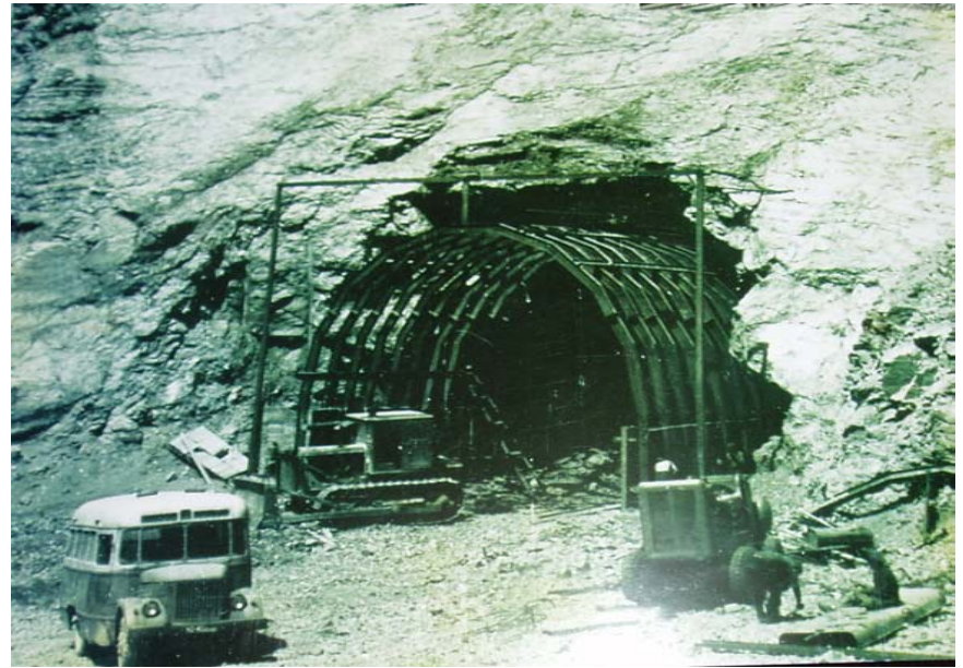
Early construction operations
